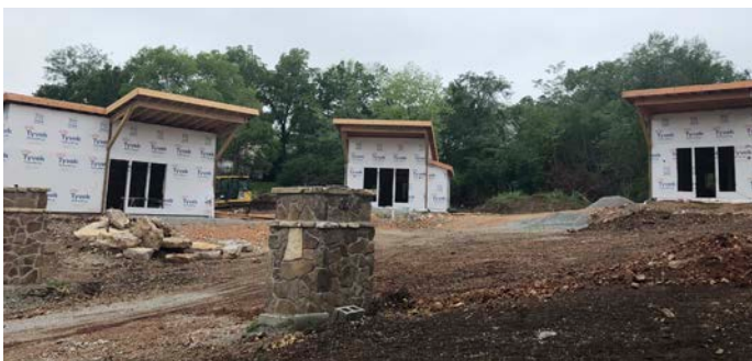
Figure 4.6: Tiny homes under construction
